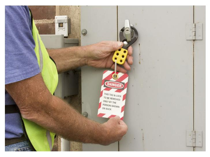
The next step is having the employee install his or her own lock and personal lockout tags on each of the disconnecting means that have been opened. Keys to the locks should be controlled rigidly so that each employee who might be exposed has confidence that the switches cannot be closed without his or her knowledge. Each employee should sign and install individual lockout tags that identify the employee and the date the tag was affixed.
