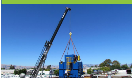
Installation of drop box furnace
