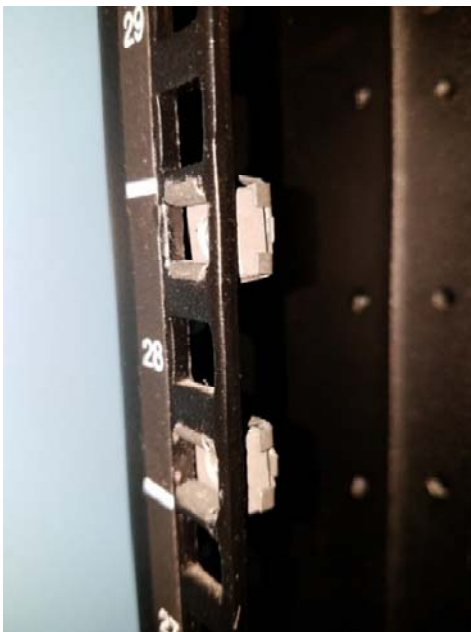
Cage nuts placed in rack rail (1RU shown) Long screws mount panel, hex nuts mount 1RU brackets
