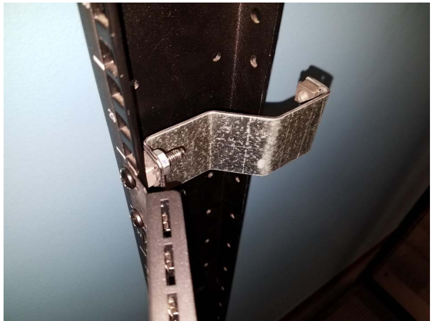
Cage nuts placed in rack rail (1RU shown) Long screws mount panel, hex nuts mount 1RU brackets
