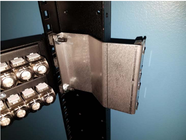
Long screws mount panel, hex nuts mount 2RU brackets
